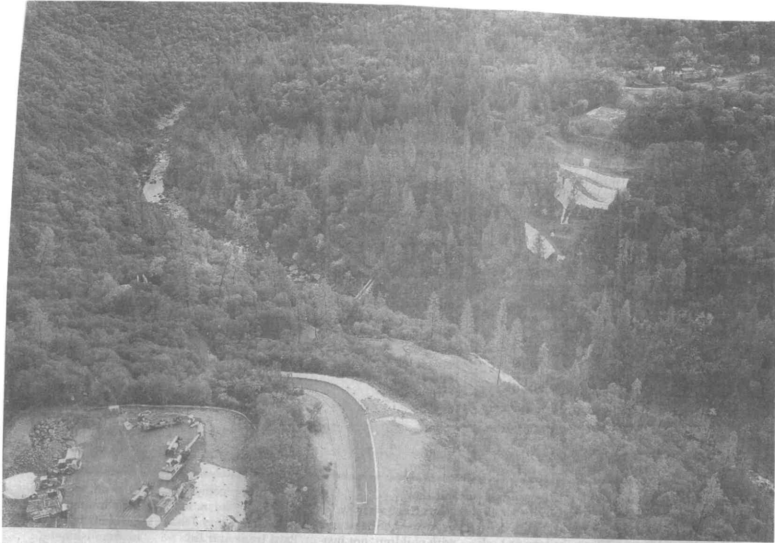
The ridgetop-to-ridgetop Mosquito Bridge project is seen from the air. The new bridge to Mosquito will rise some 400 feet over the historical bridge.
